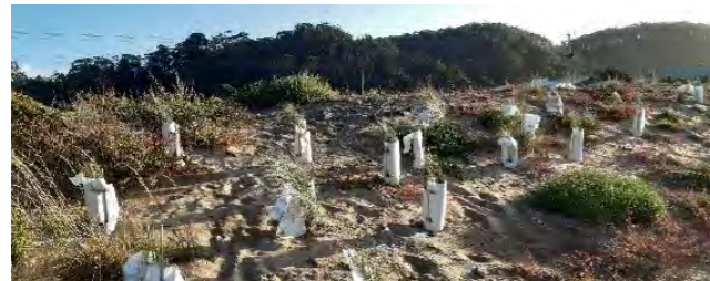
Sand placed over rock revetment and planted out with native coastal species and a section of the stabilised bank around 9 months later.
